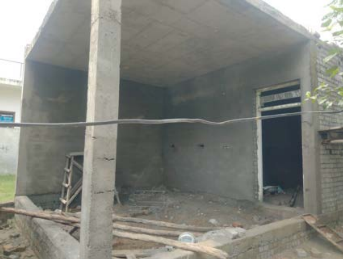
Midday meal kitchen and dining area construction is in progress at GMS Chandumajra
