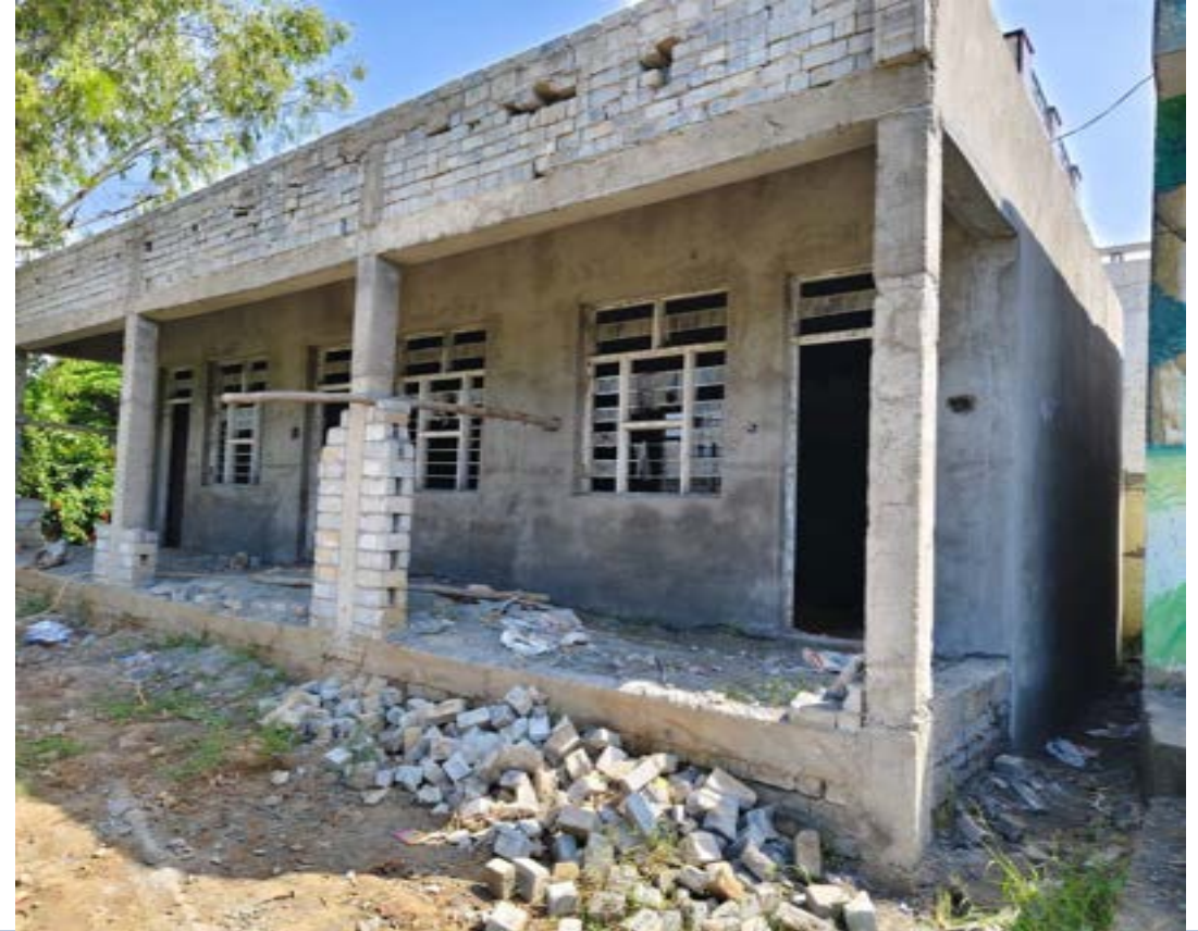
Classroom structure completed while flooring work is in progress at GES Kharola
