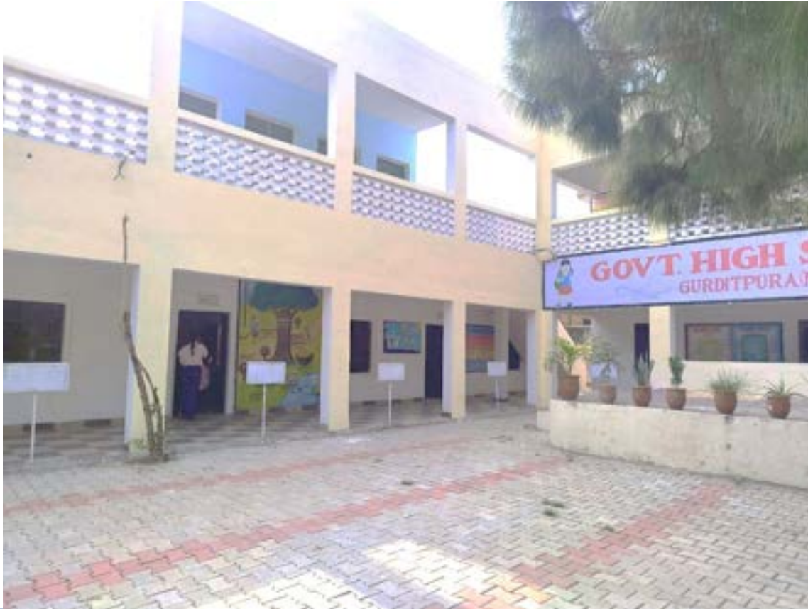
Whitewash in GHS Gurdittpura completed
