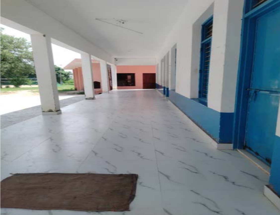
Floor tiling is in progress at GES Hariyon
