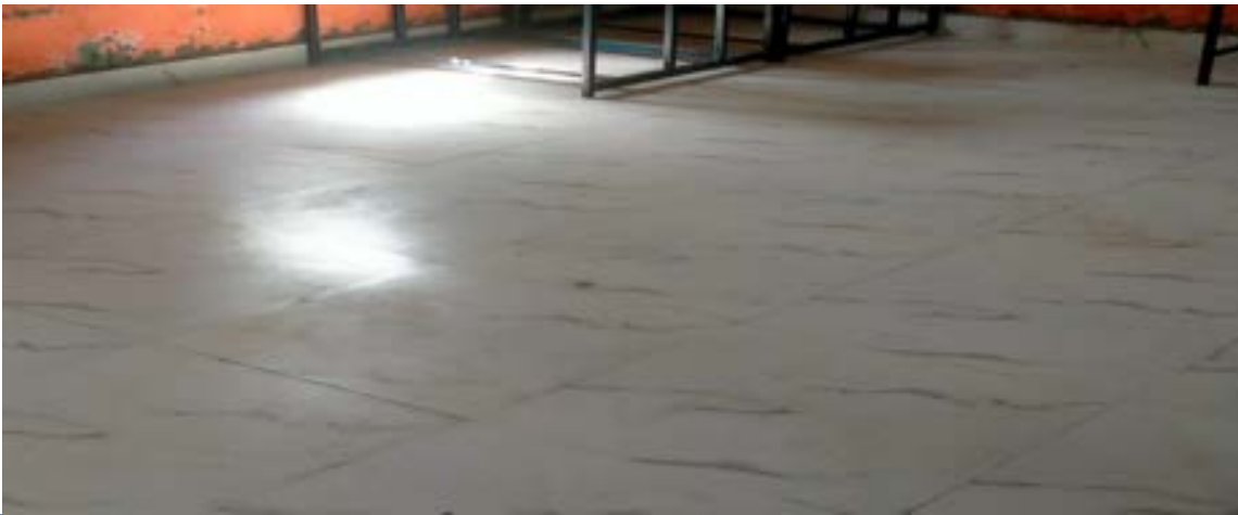
Paver work and classroom tiling in GHS Mirzapur
