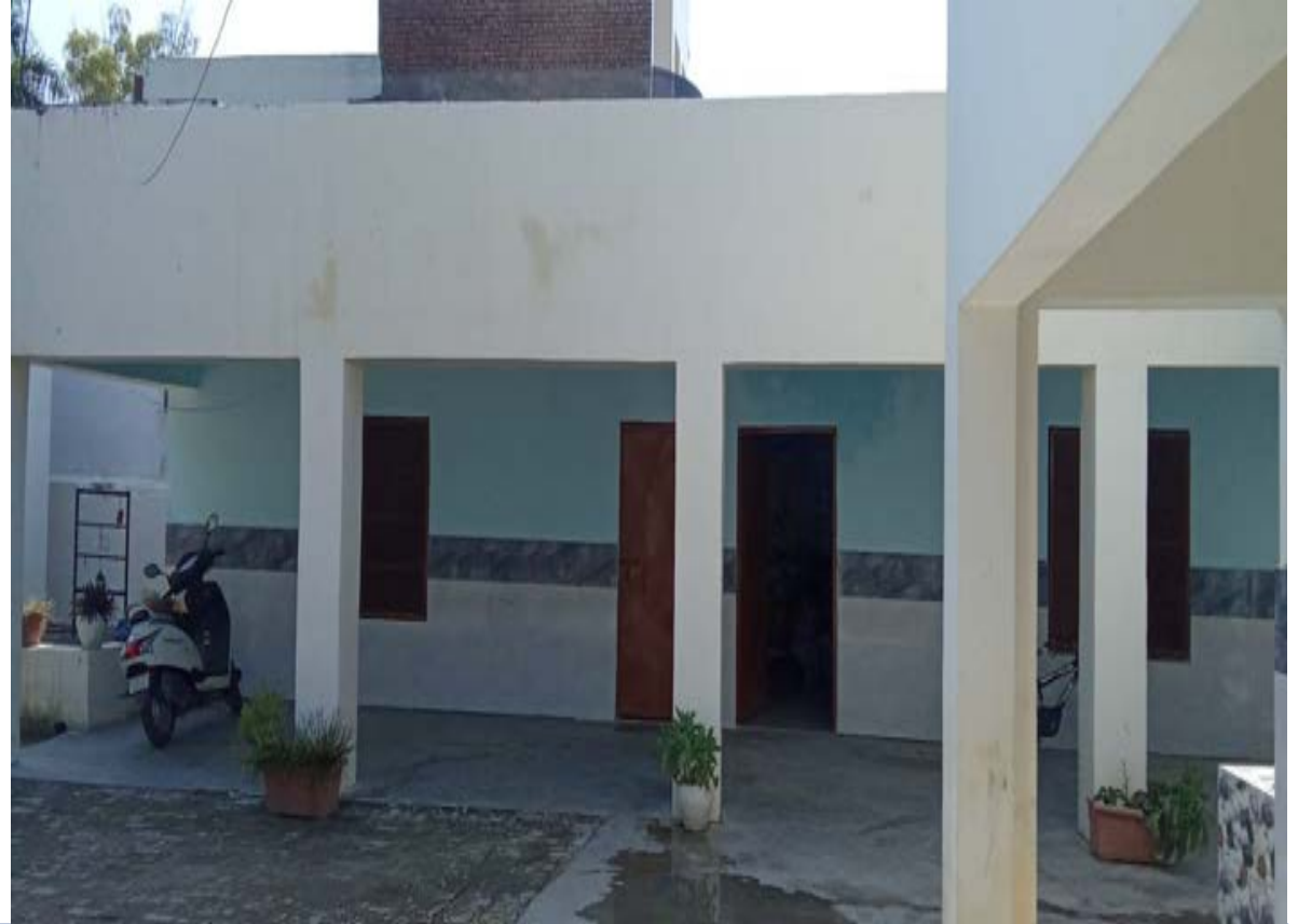
Tiling, Window Mesh and Whitewash work is in progress at GES Chandumajra
