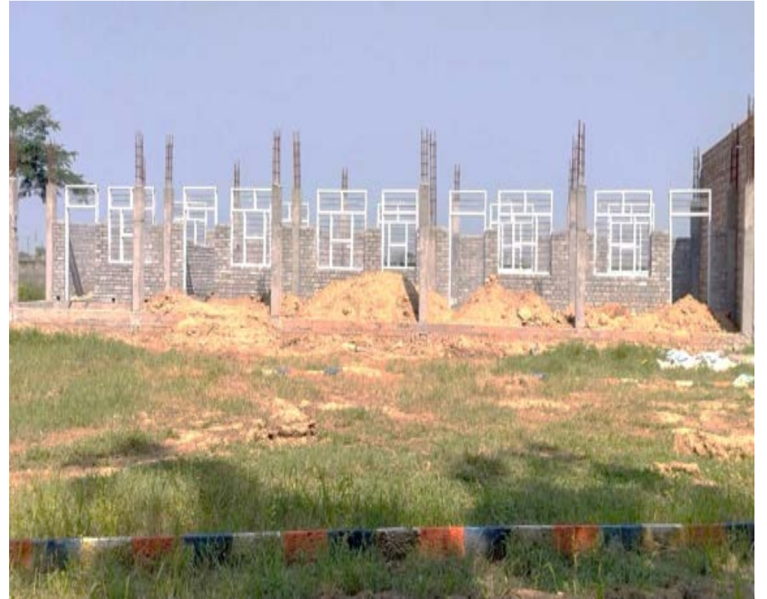
Construction of Classrooms in GES Urna is in progress
