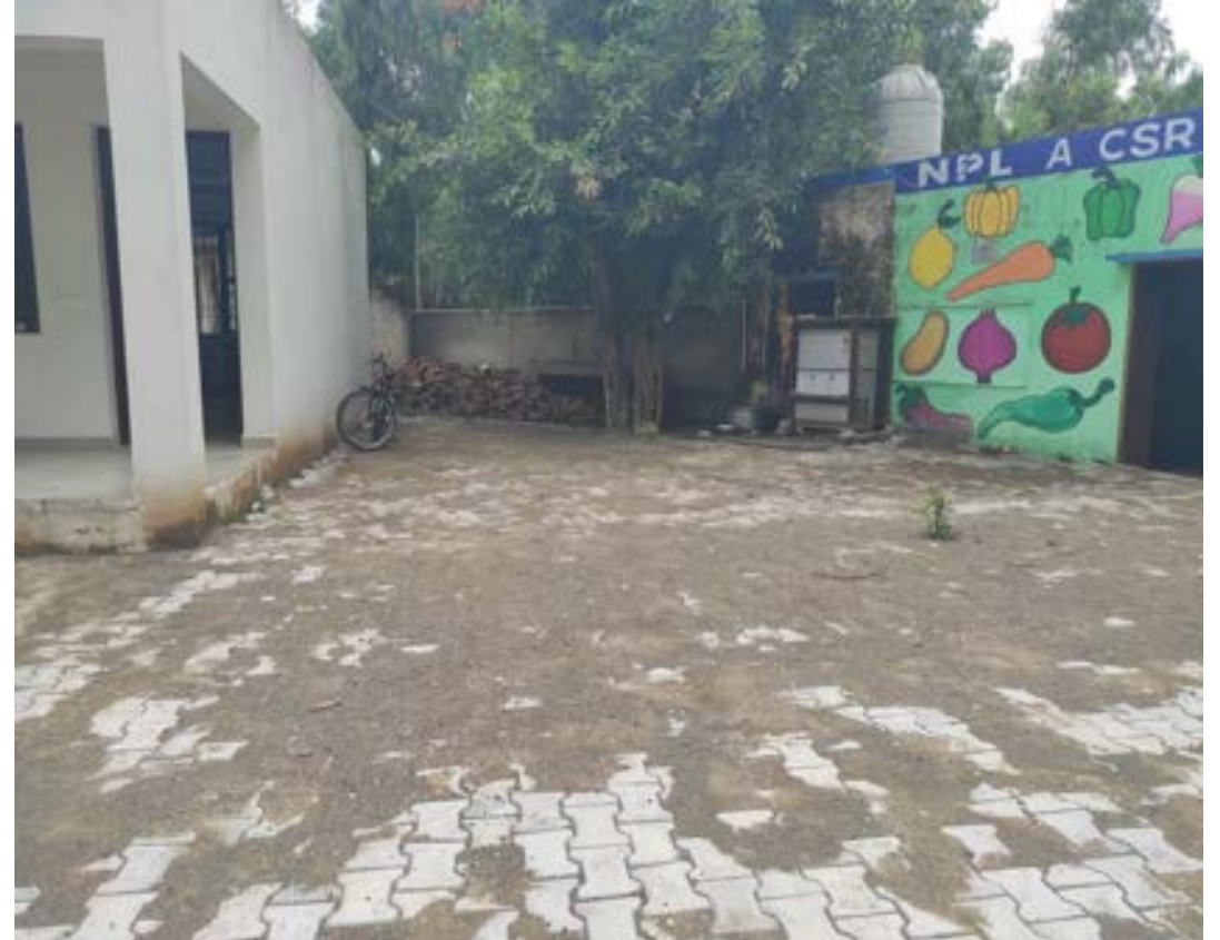
Paver work done in GES Bhagrana
