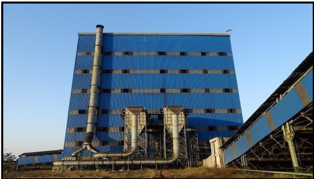
Dust Extraction System at Crusher House
