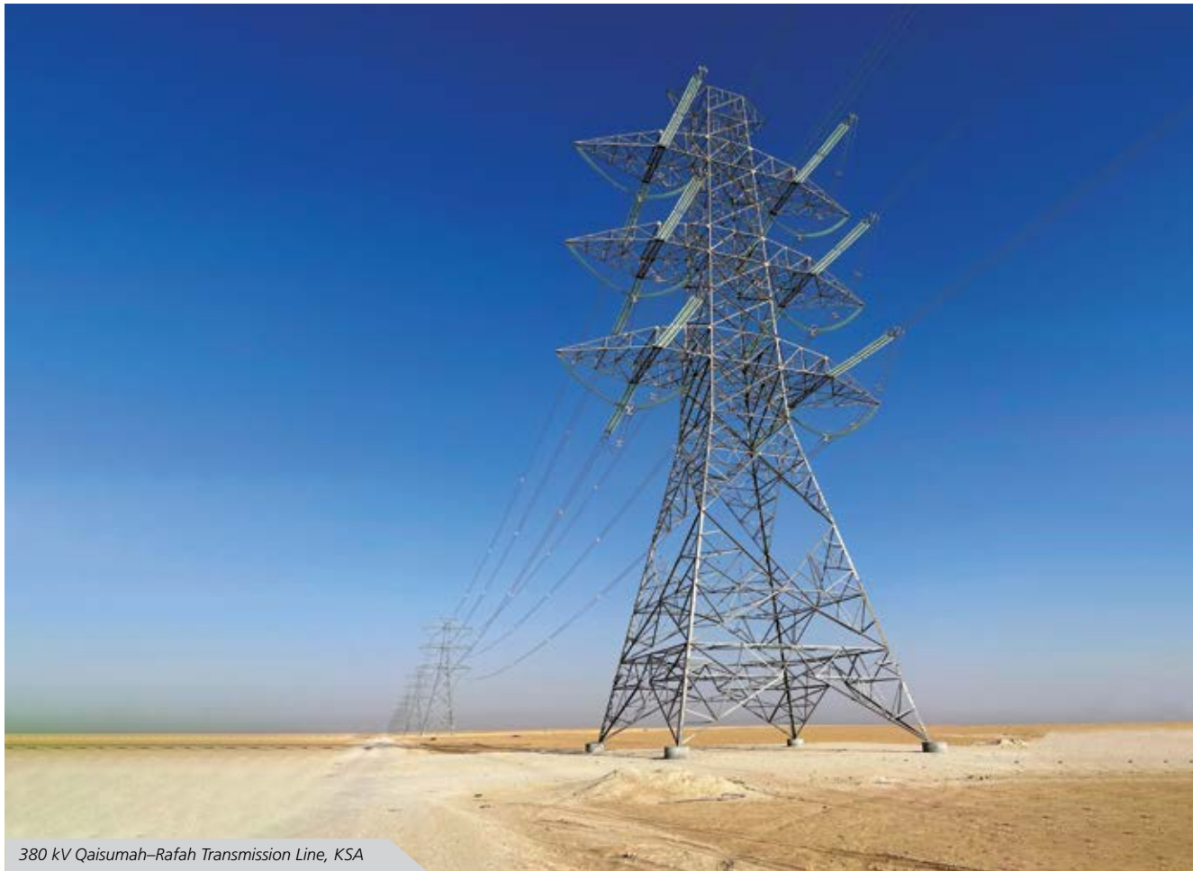
380 kV Qaisumah–Rafah Transmission Line, KSA
