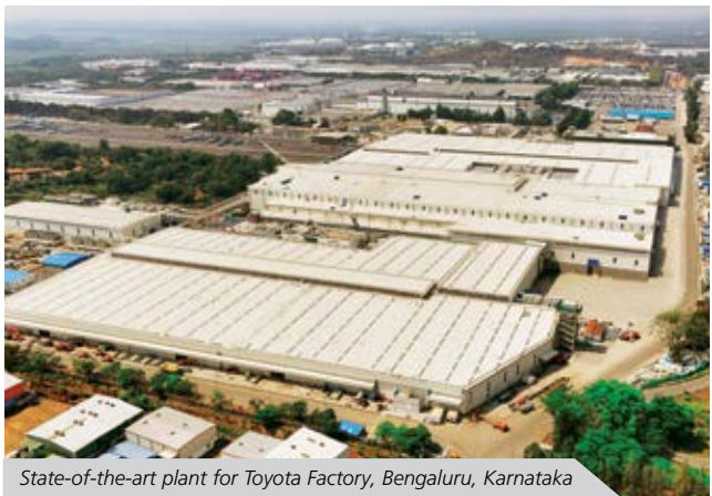
State-of-the-art plant for Toyota Factory, Bengaluru, Karnataka
