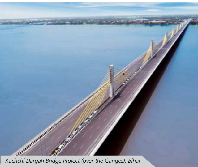
Kachchi Dargah Bridge Project (over the Ganges), Bihar
