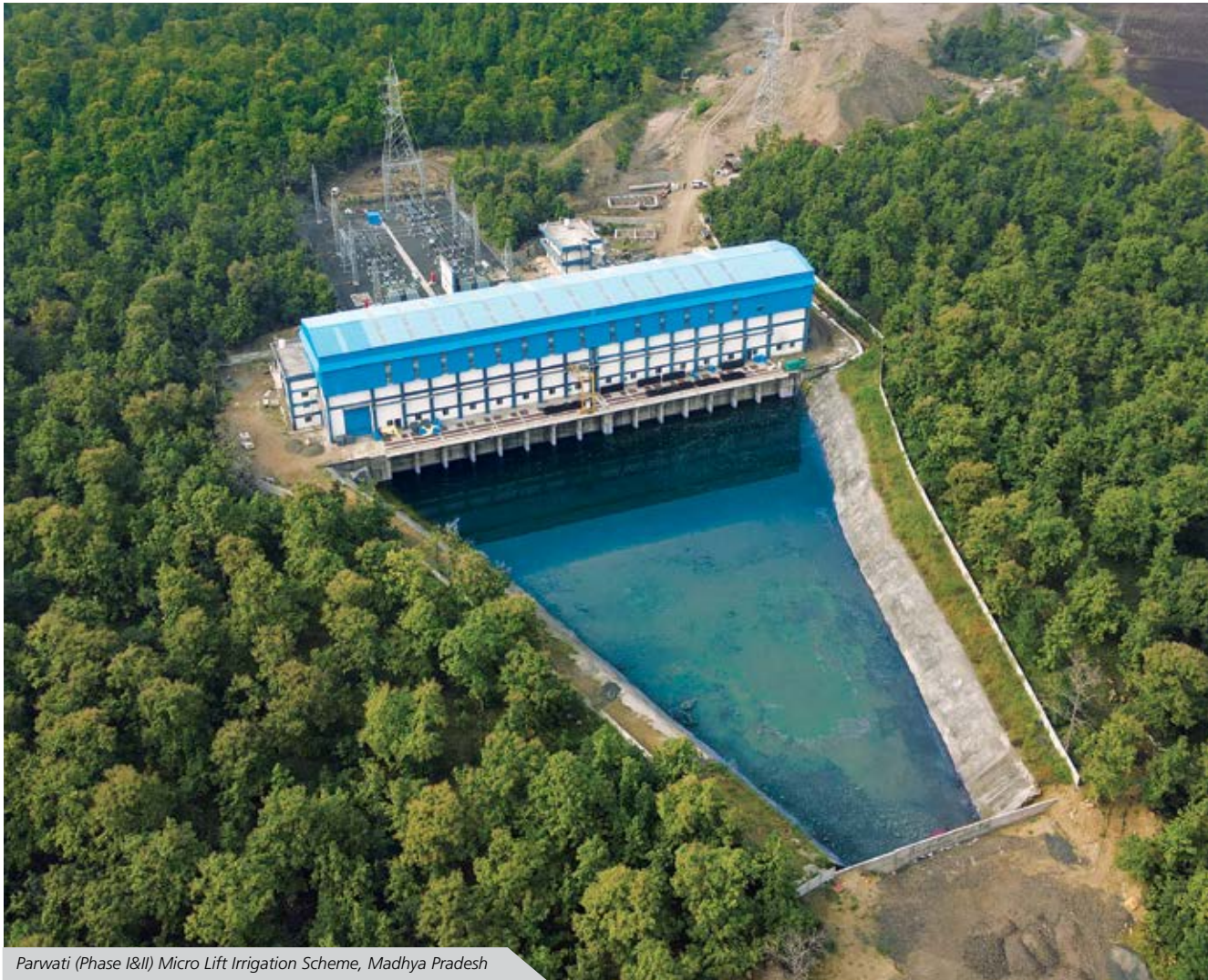
Parwati (Phase I&II) Micro Lift Irrigation Scheme, Madhya Pradesh
