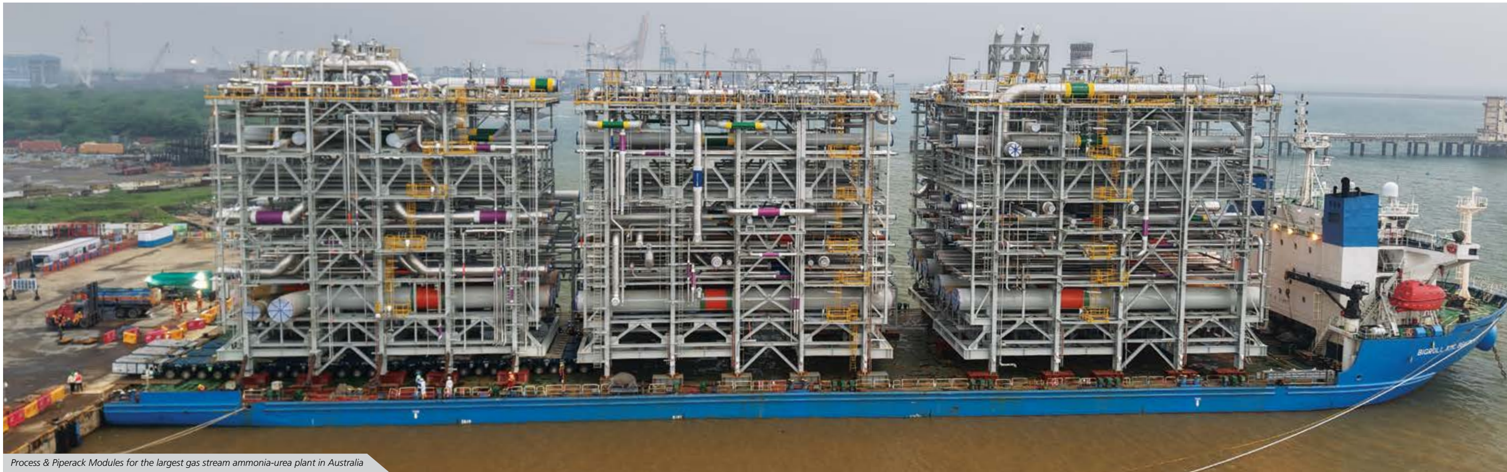
Marine Terminal Expansion Project, Juaymah NGL facilities, KSA
