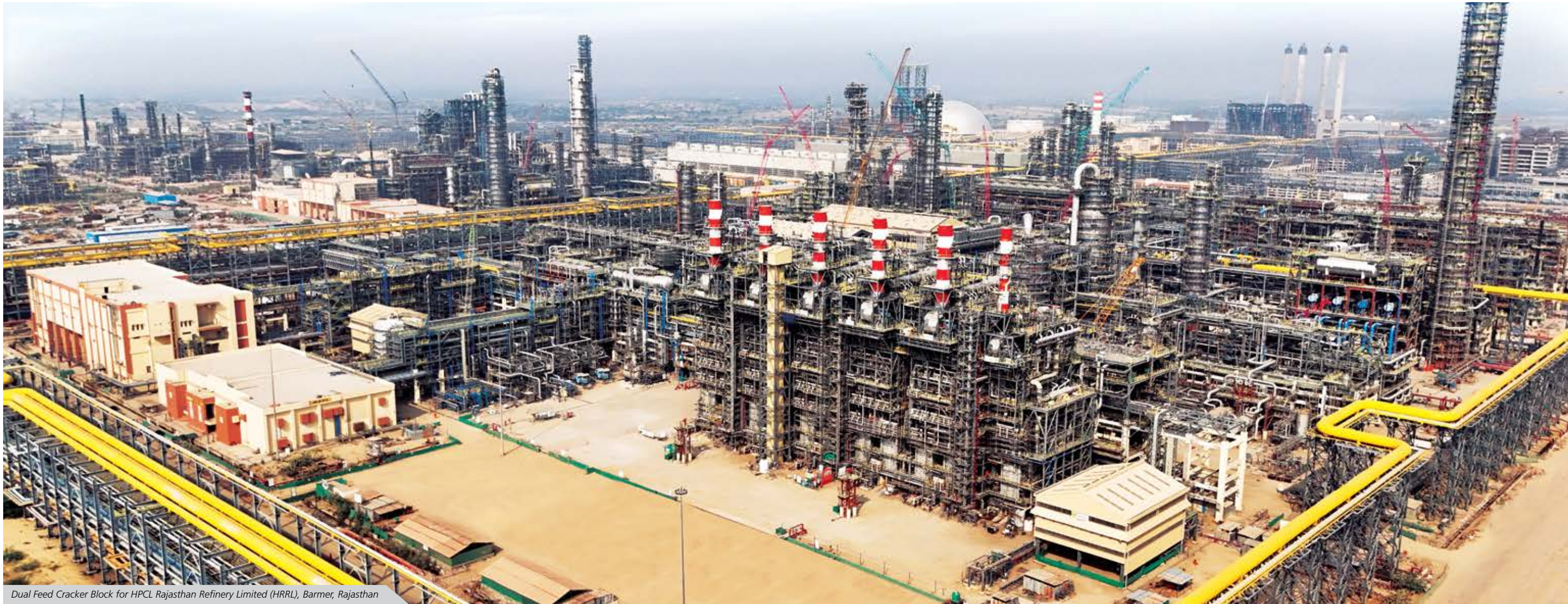
Dual Feed Cracker Block for HPCL Rajasthan Refinery Limited (HRRL), Barmer, Rajasthan
