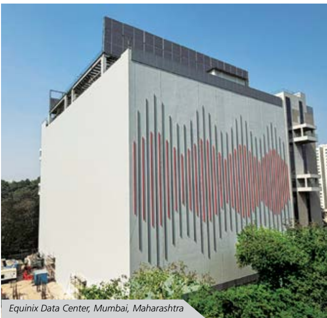
Equinix Data Center, Mumbai, Maharashtra
