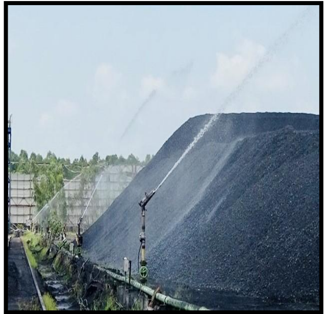
Pic-2 Dust suppression (sprinkler system) provided at each coal stockpile to arrest Dust.
