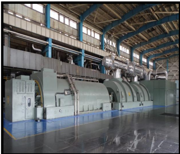
Pic-1 Acoustic enclosure provided at Turbine Generator.
