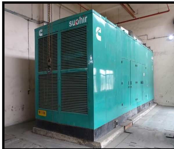
Pic-2 Acoustic enclosure provided at Diesel Generator.
