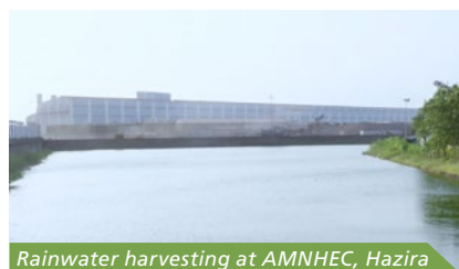
Rainwater harvesting at AMNHEC, Hazira
